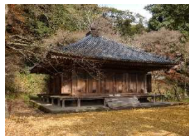
Designated Prefectural Tangible Cultural Properties (Structures) 760 buildings (as of May 1, 2022)
